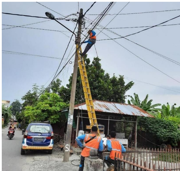
Figure 3. Medium voltage air network inspection and checking
